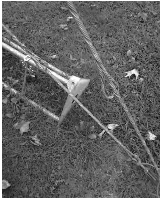
FIGURE 8 - TWIST TIES USED TO ATTACH GUYS TO HOISTING MAST
