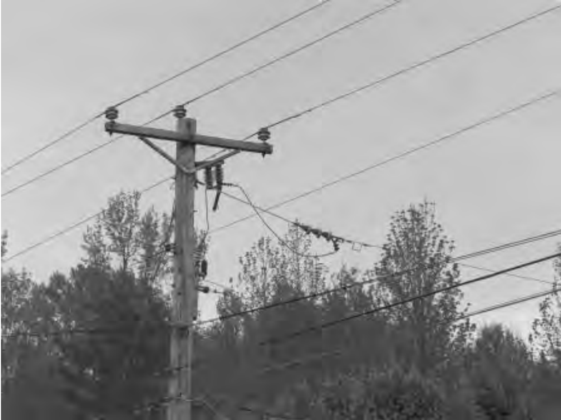
typical example of slack span
