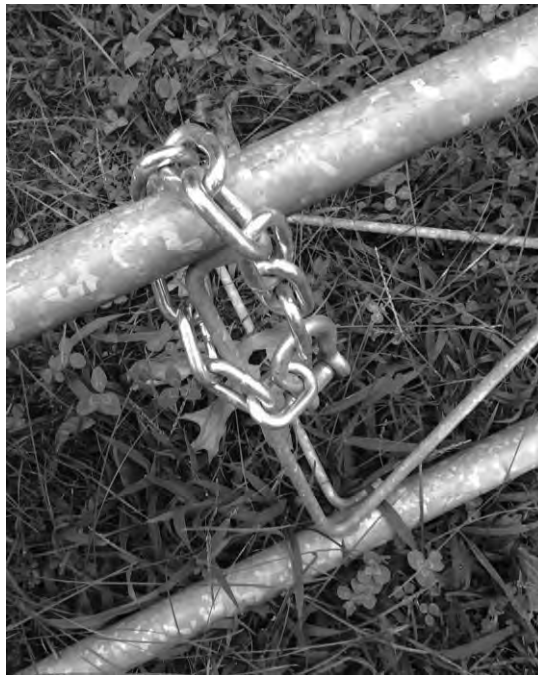
FIGURE 9 - CHAIN USED TO ATTACH HOISTING MAST TO TOWER GUYS
