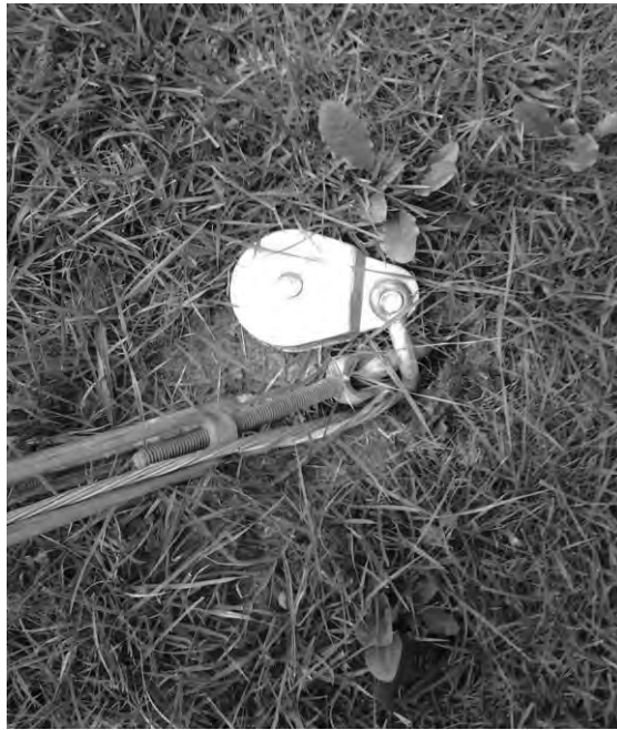
FIGURE 10 - PULLEY ATTACHED TO GUY ANCHOR USED FOR HOISTING TOWER
