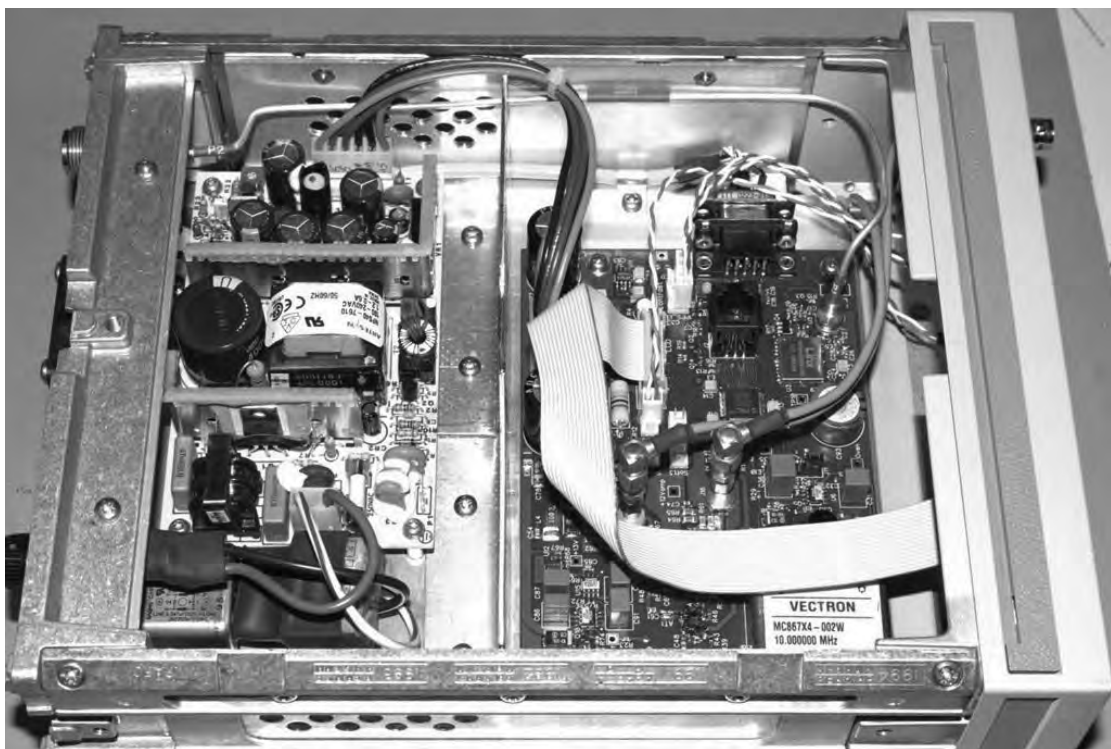
Figure 3. GPSDO board installed in the System II cabinet
