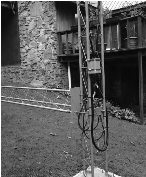
FIGURE 7 - HOISTING MAST ATTACHED TO TOWER
